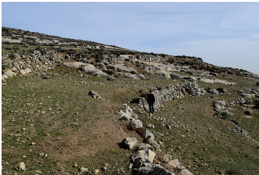
Fig. 16. Retaining Walls, Zone 1 Photo by Robert Miller.
