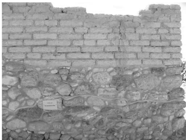
Fig. 4: Mudbrick walls with fieldstone foundations and lower wall. Photo by Ian Scott, creative commons.
